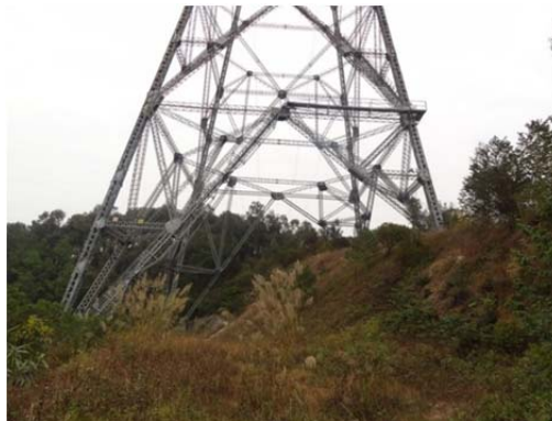
Fig.1 Natural slopes on the tower legs
